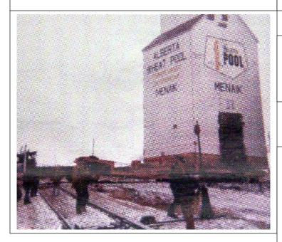
Moving day for the Menaik elevator in March 1978. It took movers three hours to transport the structure five kilometers.
